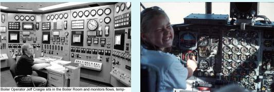
Boiler Operator Jeff Craigie sits in the Boiler Room and monitors flows, temperatures and pressures of the boilers and feed-water system. Photo by Ryan Solomon
